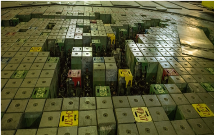
Control rod coverings for the nuclear reactor in Chernobyl's Unit 1. Source: RadioFreeEurope
