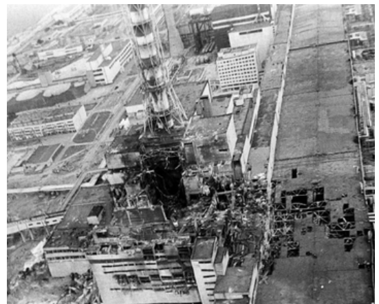
The remains of the Chernobyl nuclear power plant after the explosion. Source: Associated Press
